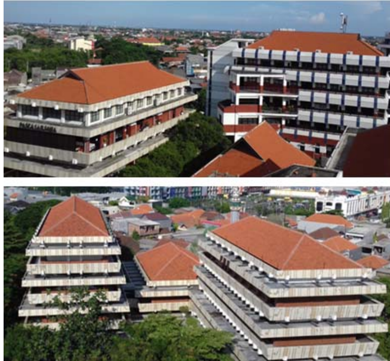
Fig. 2. Gabled roof (upper) and Hip roof (lower) types of University of Surabaya buildings
