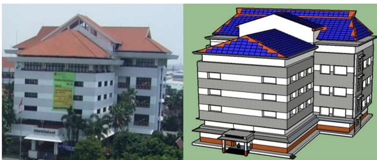
Fig. 3. Library building as representative building used in simulation
