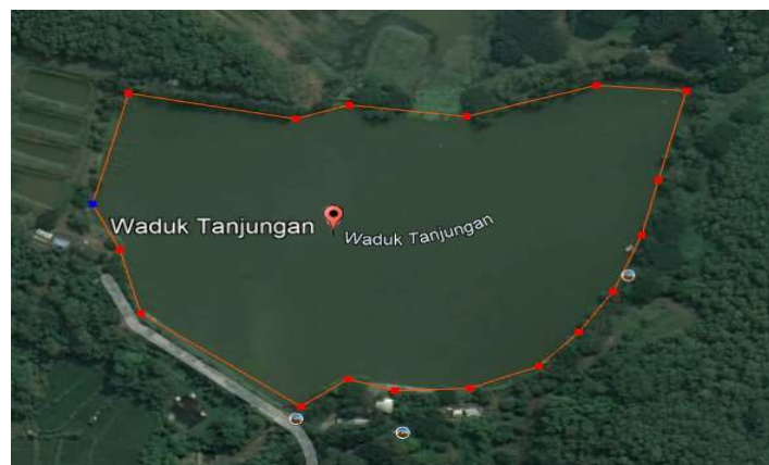
Fig 1. Fig 2. Tanjungan Dam on Google Earth view
