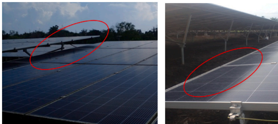
Fig. 8. Shading caused by the PV system itself.
