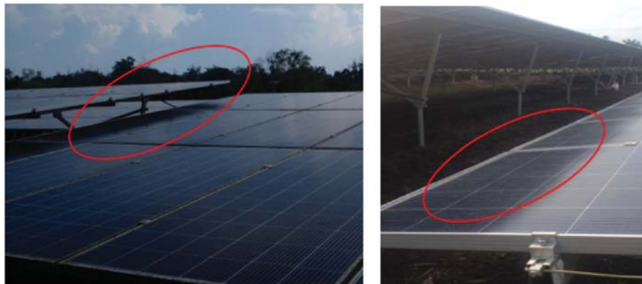
Fig. 8. Shading caused by the PV system itself.
