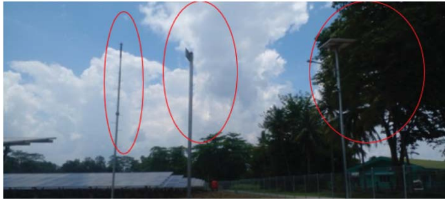
Fig. 7. Potential shading caused by surrounding objects on the PV system.
