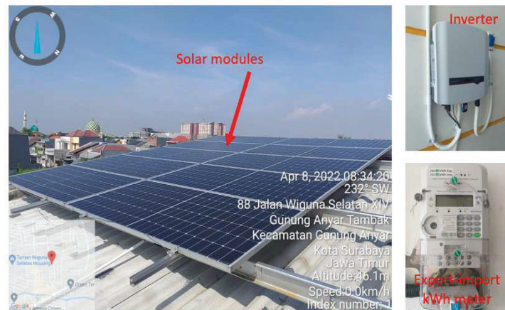
Figure 2. Solar modules, inverter, and export-import kWh meter
